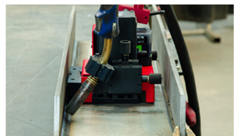
Welding in narrow spaces
